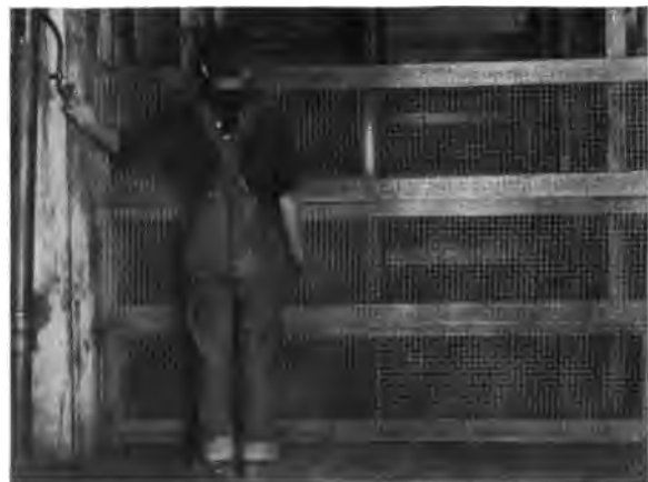
Fig. 5. Telescoping Elevator Gate, for use where there is limited Head-Room.*
